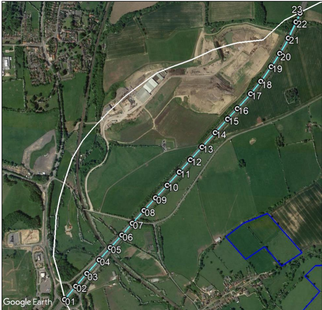
Figure 5 A1(M): road receptors 01 to 23 – aerial image
